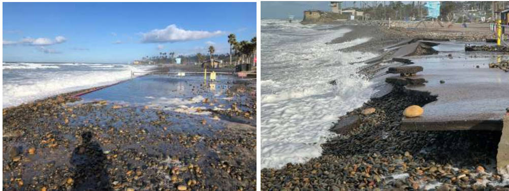
Photos 3 and 4: Erosion and storm damage of Cardiff State Beach with lot closures in January and February. Provided by CA State Parks.
