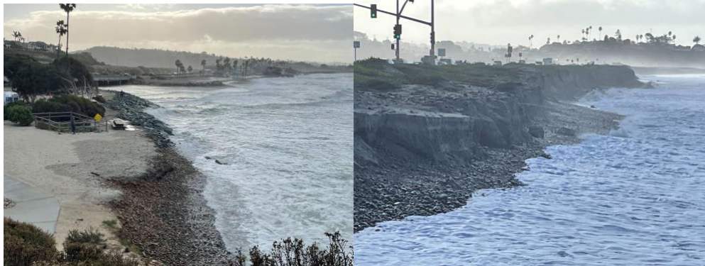
Photos 1 and 2: Erosion and storm damage of Swamis 3b and 4. Showing lack of beach access in January and February. Provided by CA State Parks.
